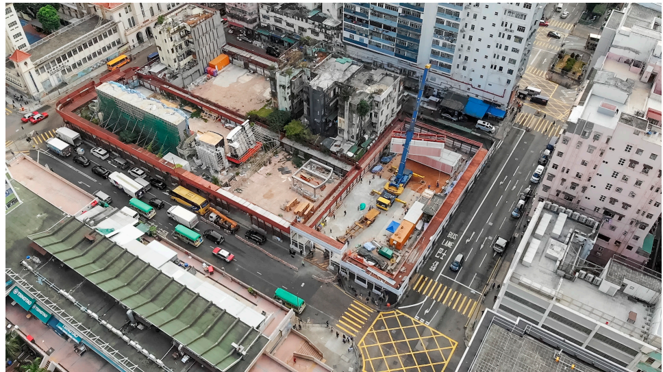
Figure 1. Construction of NC220 (source: https://www.socialhousing.hkcss.org.hk/en/node/58 , accessed on 2 July 2023).
