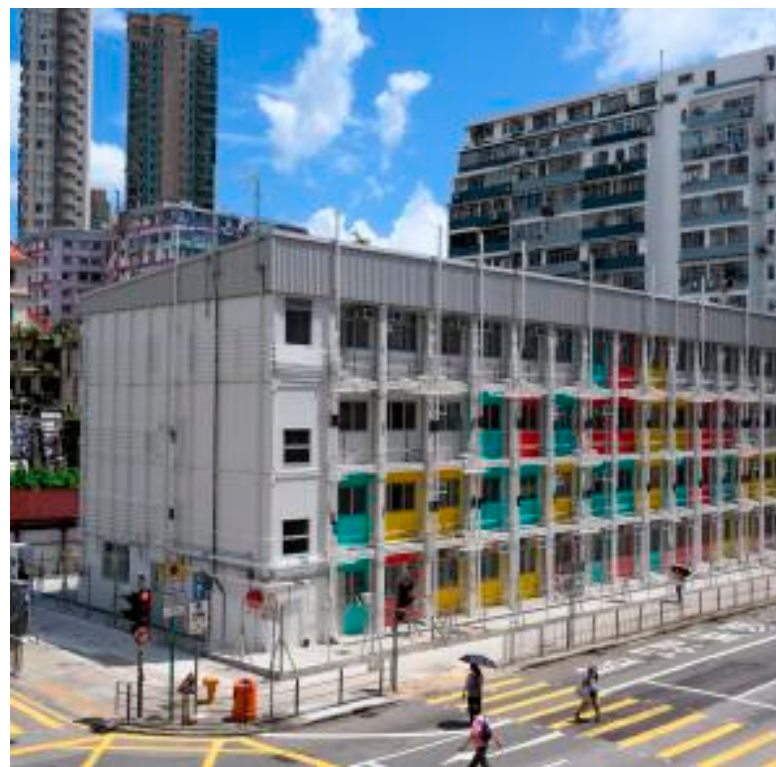
Figure 2. NC220 building (source: https://www.socialhousing.hkcss.org.hk/en/node/58 , accessed on 2 July 2023).
